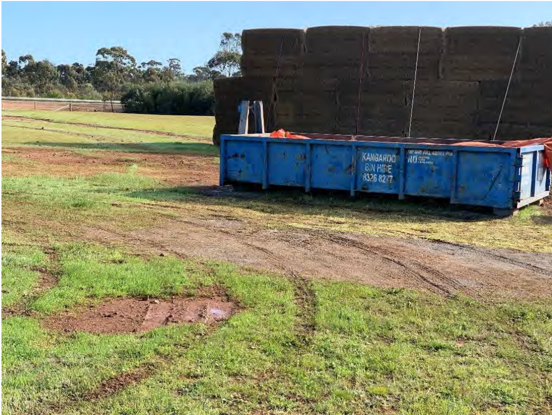
Figure 14. Kapunda drill site minutes after the drilling crew demobilised with the waste skip waiting for collection.
