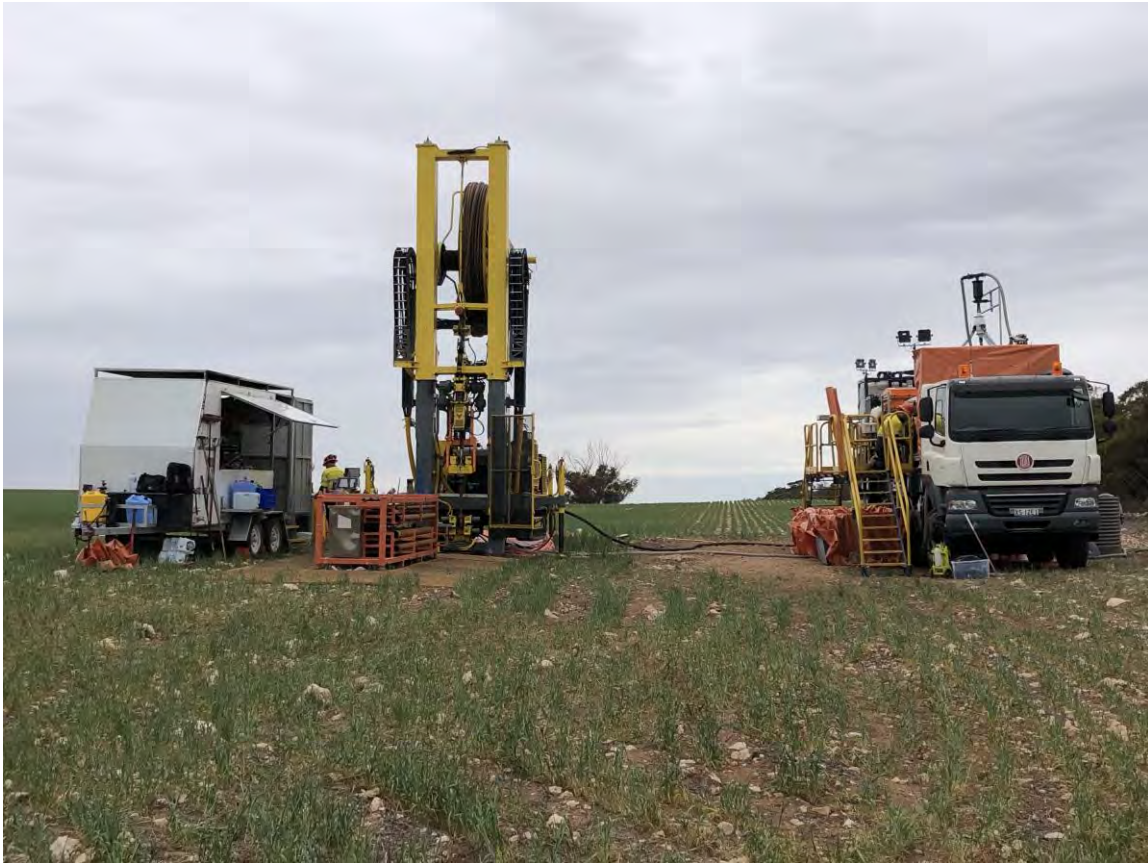
Figure 15. Delamerian South (Alawoona) drill site in corner of wheat paddock. This drill site layout utilising two skips to collect solid waste.
