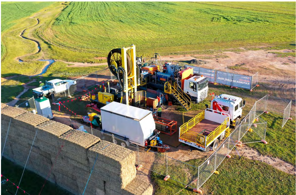
Figure 13. Aerial view of the Kapunda drill site.
